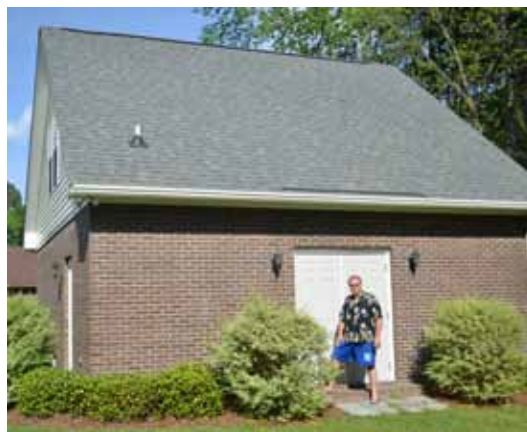
Completed in August 2007, it took a year to plan and seven months to build the Shealy's percussion studio. Mom Vickie Shealy's crafts studio occupies the entire second floor.
